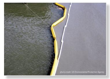
Environmental engineering controls such as turbidity silt curtains are highly effective means to contain and control dispersal of contaminants during wet dredging.
